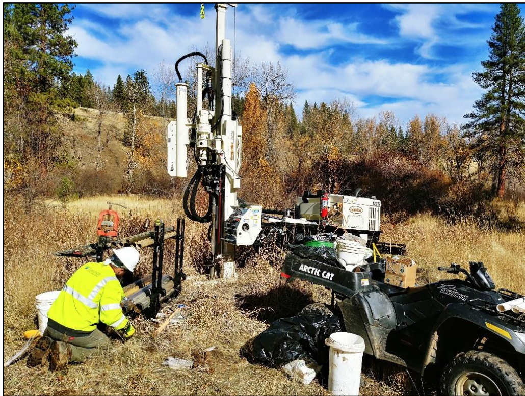
FIGURE 13 INSTALLATION OF GROUNDWATER WELL #21
